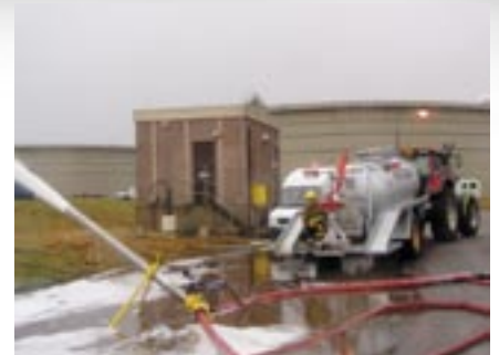
Water from the high pressure mains may be piped through the monitor on the rear of the tanker or the foam chemical can be piped to free standing monitors as here.
