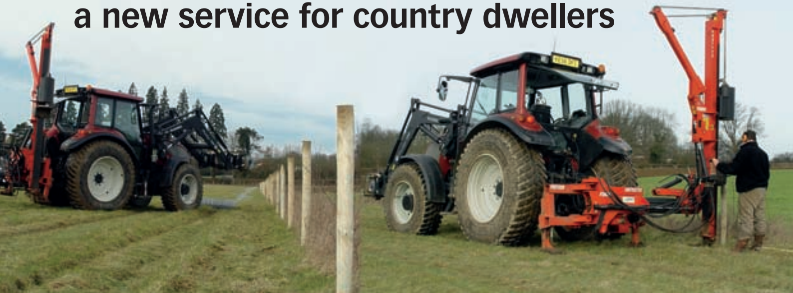
With post driver on the rear and stakes and wire on the loader there is little reason for other machines to come onto the land. James' M120 fitted with a loader and grassland tyres is ideal for fencing work
